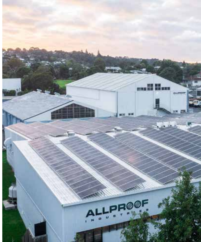
Allproof recently completed a large solar installation on the roof of its main production facility on Auckland's North Shore. The solar panels cover an area of 1700sq m, generating 750kWh of electricity per day and saving 49 tonnes of CO 2 from entering the atmosphere annually.
