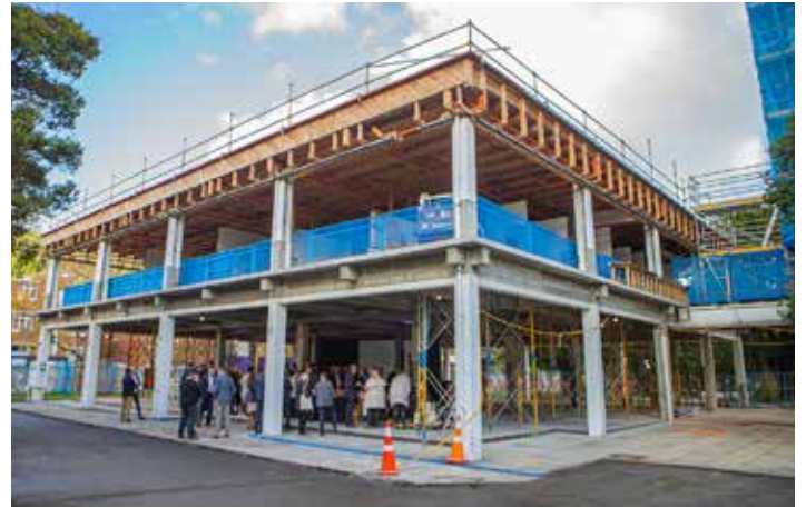
The under-construction Buddle Building, Stage 1, Blue Mountains Campus in Upper Hutt.
