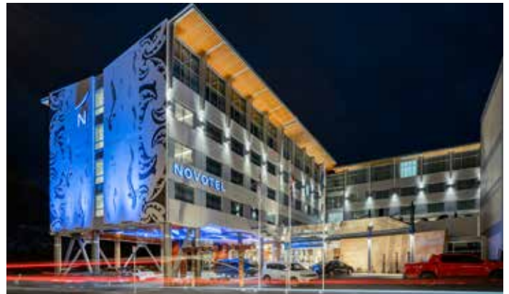
The stunning four-level extension to the Novotel Tainui Hamilton Hotel received a Gold Award at the New Zealand Commercial Project Awards 2022.
