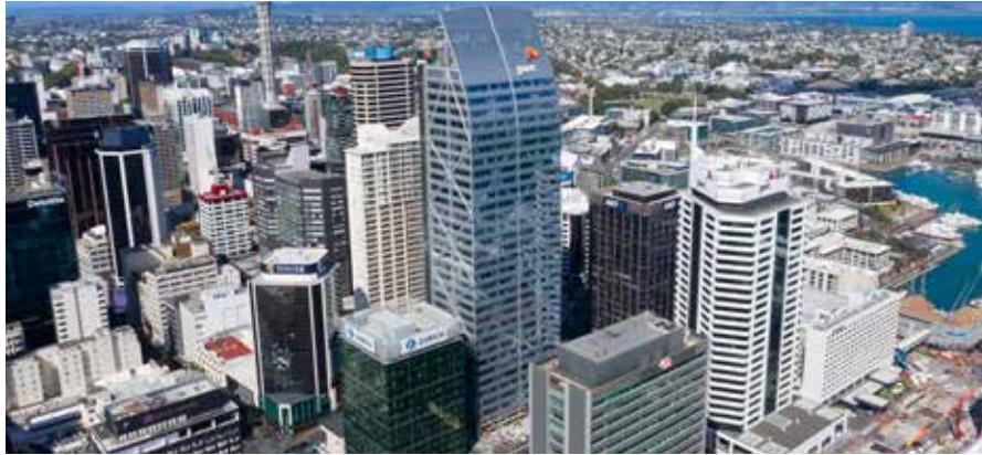
Precinct's PwC Tower in downtown Auckland was awarded a 5 Green Star rating recently.
