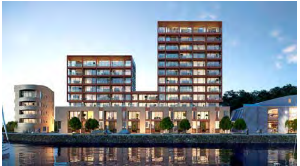
The Catalina Bay Apartments are now under construction at Hobsonville Point in Auckland.
