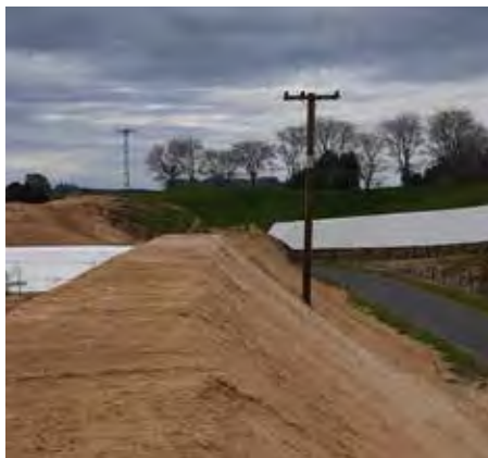
An example of where land has been recontoured an unsafe distance from existing power lines.
