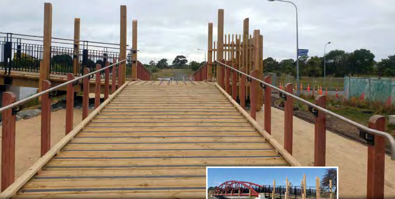
Avondale Bridge, Christchurch
