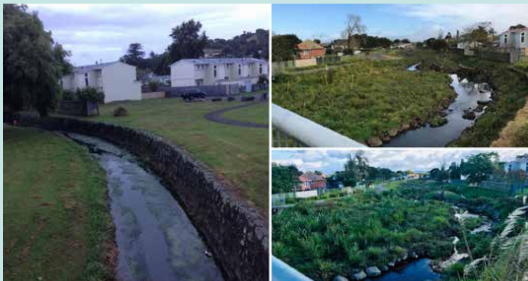
The Te Auaunga Project in Wesley, Auckland. These pics show the same spot in Feb 2016 (before), July 2018, and April 2019.
