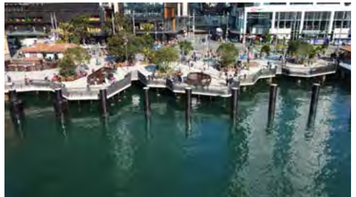
Downtown Infrastructure Development Programme, Auckland.
