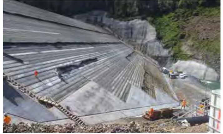
Waimea Community Dam, Tasman District.
