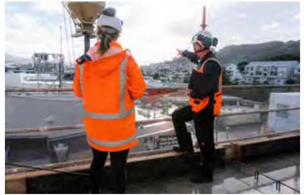
The outer layer of all winter clothing should be hi-vis, rain and wind-proof, and allow for easy opening and removal.
