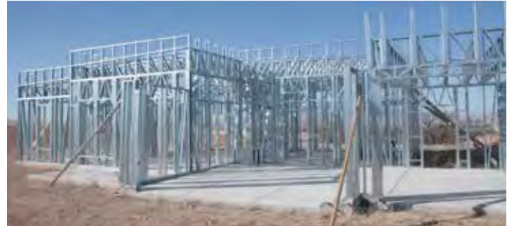
Cold-formed steel framing offers superior durability, stability, and resistance to environmental factors.
