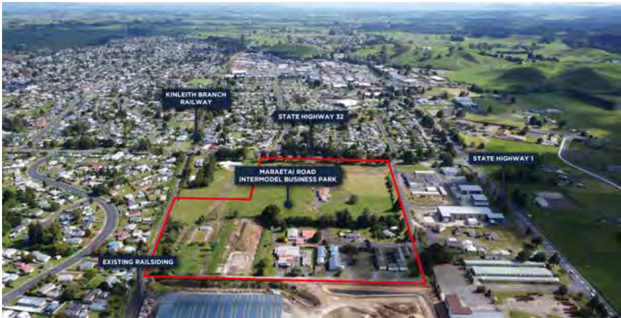
Development of the Maraetai Road Intermodal Business Park in Tokoroa will start this year, with further staged development through to the end of 2024.
