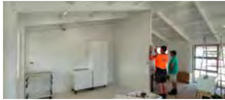
Interior work underway.
