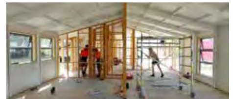
Enclosed after four days on site.
