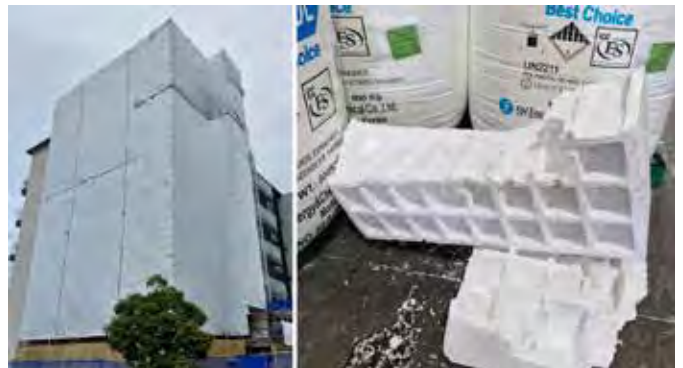
Figure 2: Left: Shrinkwrap is recycled back into builders’ polythene film (DPM). Right: Polystyrene back into polystyrene.
