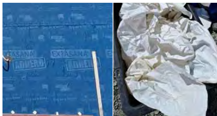
Figure 4: Left: Building paper. Right: Backing product of building paper (silicon-based).
