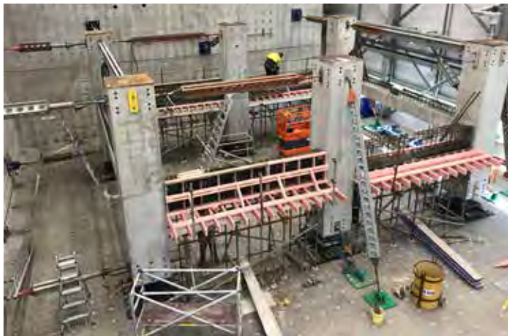
The ReCast team developed and tested retrofit solutions aimed at strengthening precast concrete hollow-core floors.
