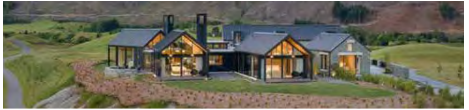
This entry by Master Stroke, winner of the Southern Region New Home over $4 million category, is one of the Top 100 homes to go forward to a second round of judging in the 2025 Master Builders House of the Year competition.
