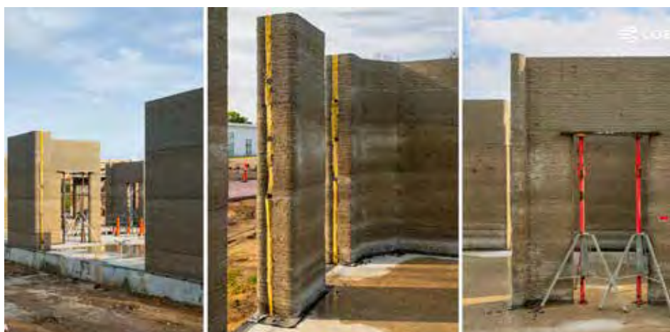
3D-printed walls of the Skovsporet ("The Forest Trail") apartments in Holstebro, Denmark.
