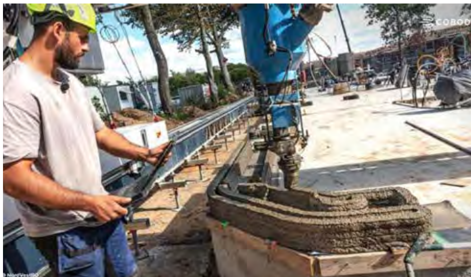
3DCP Group controls the Cobod BOD3 printer on-site. The BOD3's ground-based track system allows uninterrupted printing for long wall sections, achieving consistent results with a three-person team.
