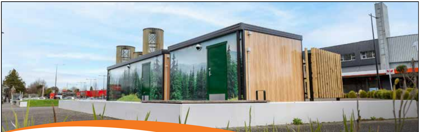
Pictured above: South Waikato District Council Bathroom Blocks for Tokoroa township
