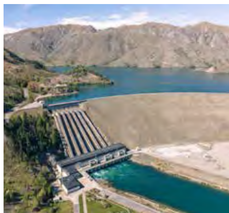
Benmore Hydro Station in Canterbury is undergoing a $65 million seismic upgrade.
