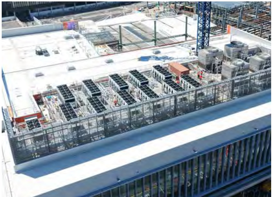
Each of the industrial heat pumps is roughly the size of a shipping container, and delivers up to 600kW of heating or cooling, around 100 times the output of a typical home unit.
